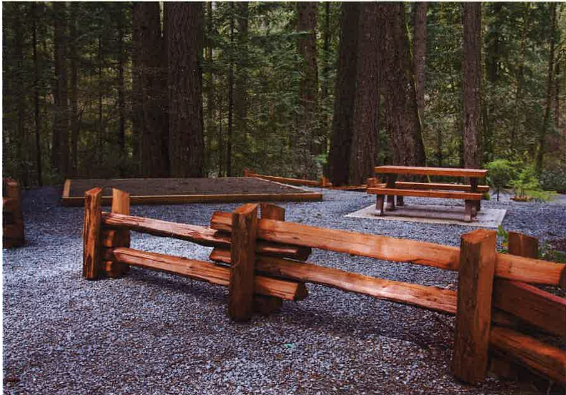
Figure 7 Example of Split Rail Fencing at Campsite from Goldstream Provincial Park.
