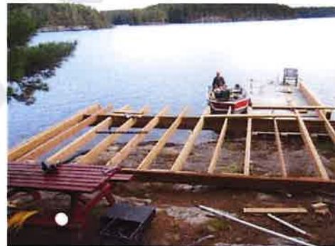
Figure 5 Example of Wood Decking Construction.
