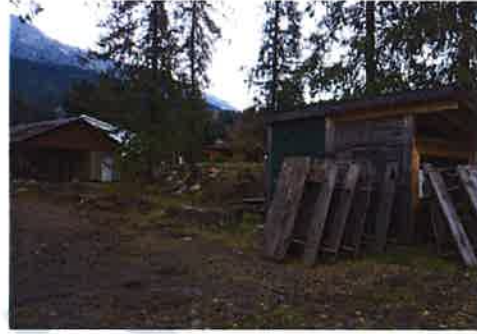
Figure 1 Existing Buildings at Lakeside Campground.
